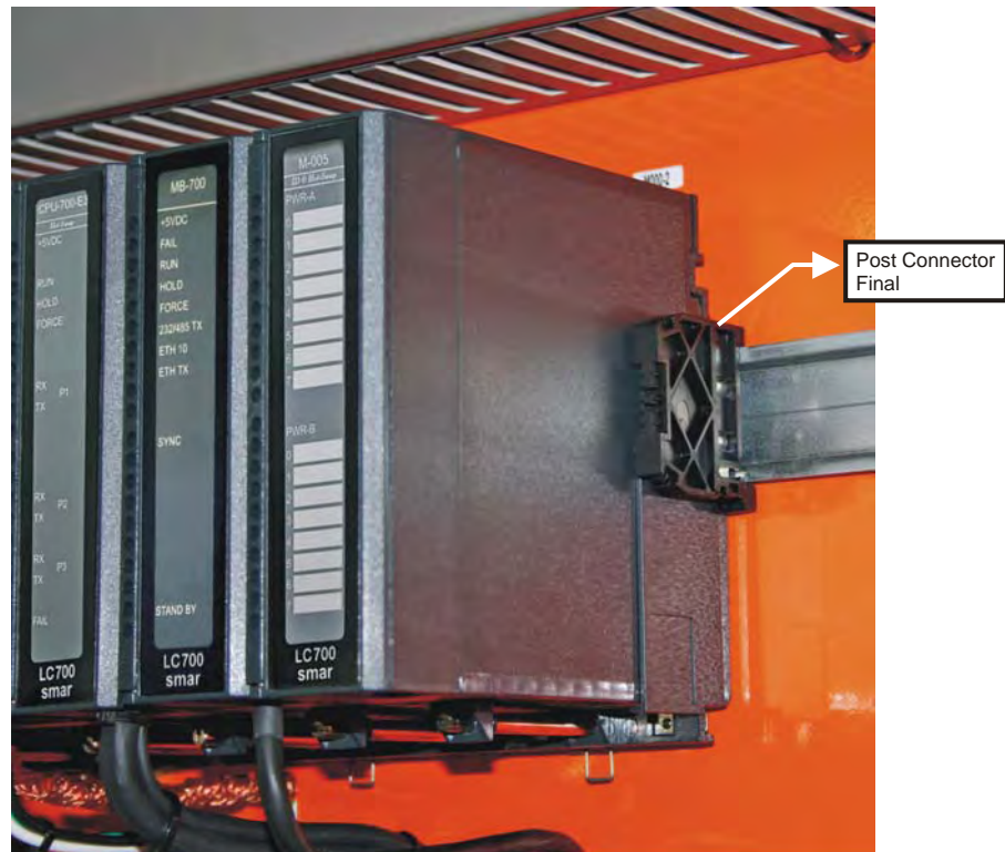
Figure 4.3 – Final Post that Holds the Racks on the Rail
