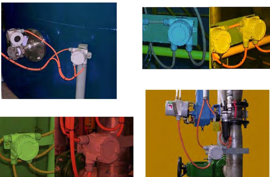
Figure 1.14 –Field Network with Derivation Box
