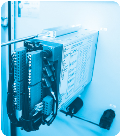
Figure 2 shows the screwdriver and the fixing clip bolt of the CD600 Plus (back view of the panel)
